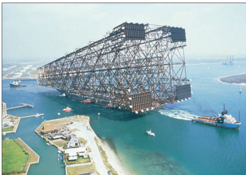
Figure 1. Steel jacket being towed to offshore waters for establishment of an offshore rig.
