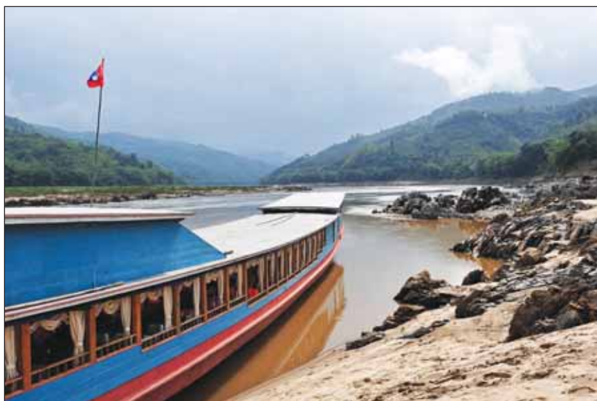
Figure 5. Site of the proposed Xayaburi Dam on the Mekong mainstream, Laos.
