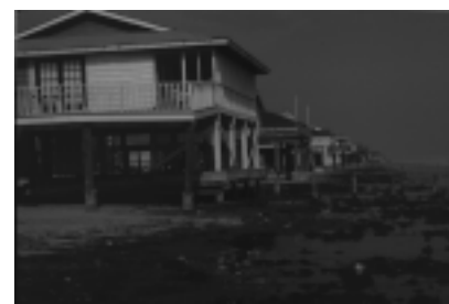
FIGURE 35 Erosion Damage from Tropical Storm Frances (1998)
