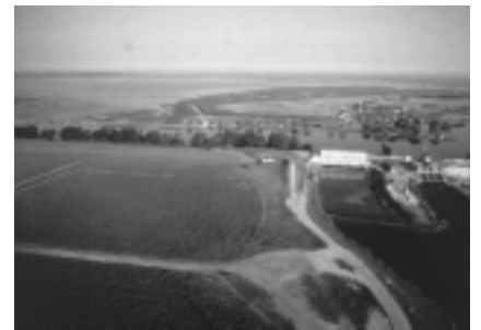
FIGURE 2 Water Control Structure
